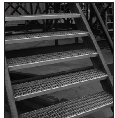
Stringer firmly anchored to floor by bolts
