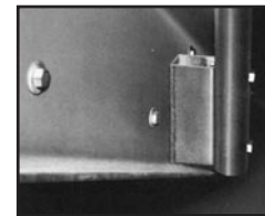
Bolted handrail attachment
