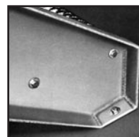
Stringer firmly anchored to floor by bolts
